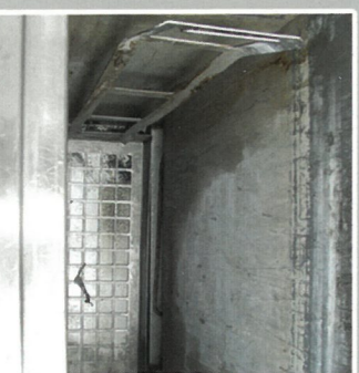
Rinse tank with hot water ensuring it is empty.
